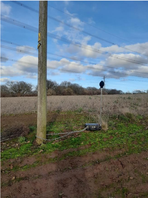
Plate 14.2-69 Equipment Photos NML24 - 2026
