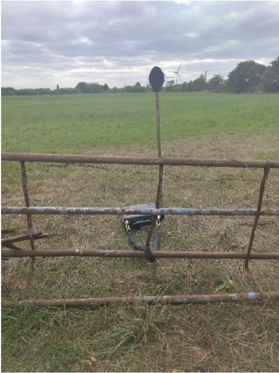
Plate 14.2-25: Photos of Equipment at NML11
